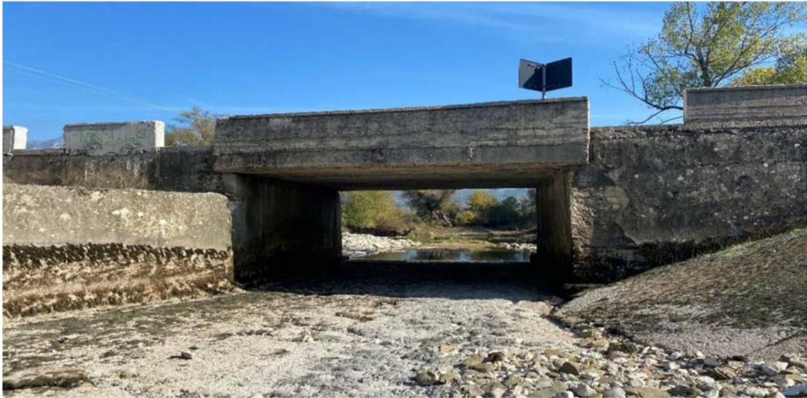
Existing Viroi Bridge
